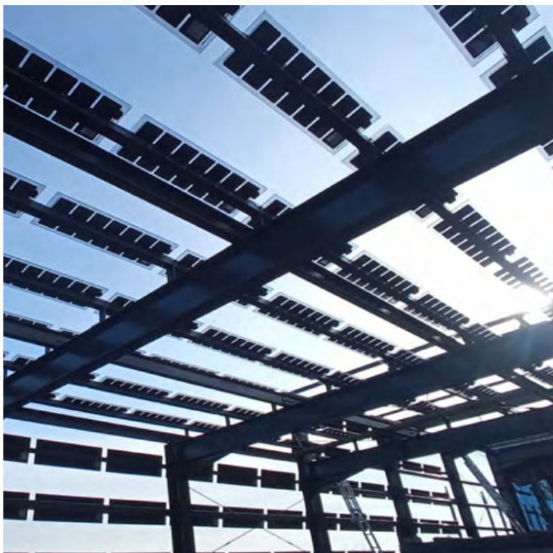
AluClear products: BIPV Sunshades – modules in glass-glass technology
