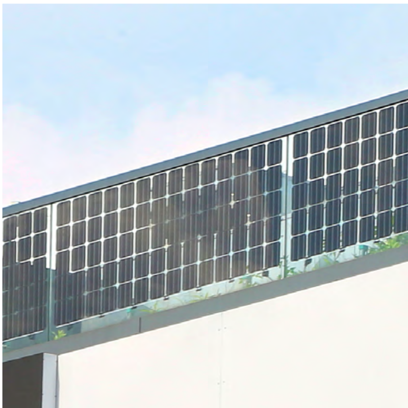
AluClear products: BIPV Balustrade with semi-transparent modules in glass-glass technology
